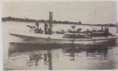
The Turnabout Torpedo Boat, named GORDON. She carried two torpedoes in a revolving gun on either side and a 6 inch Nordenfelt gun on the mainmast.
